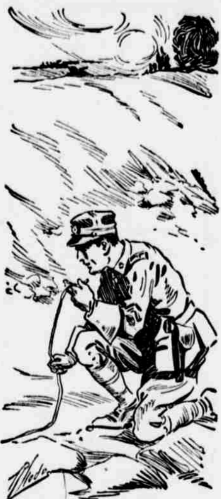
An Insulated Telephone Wire at the Bottom of a Crater.
