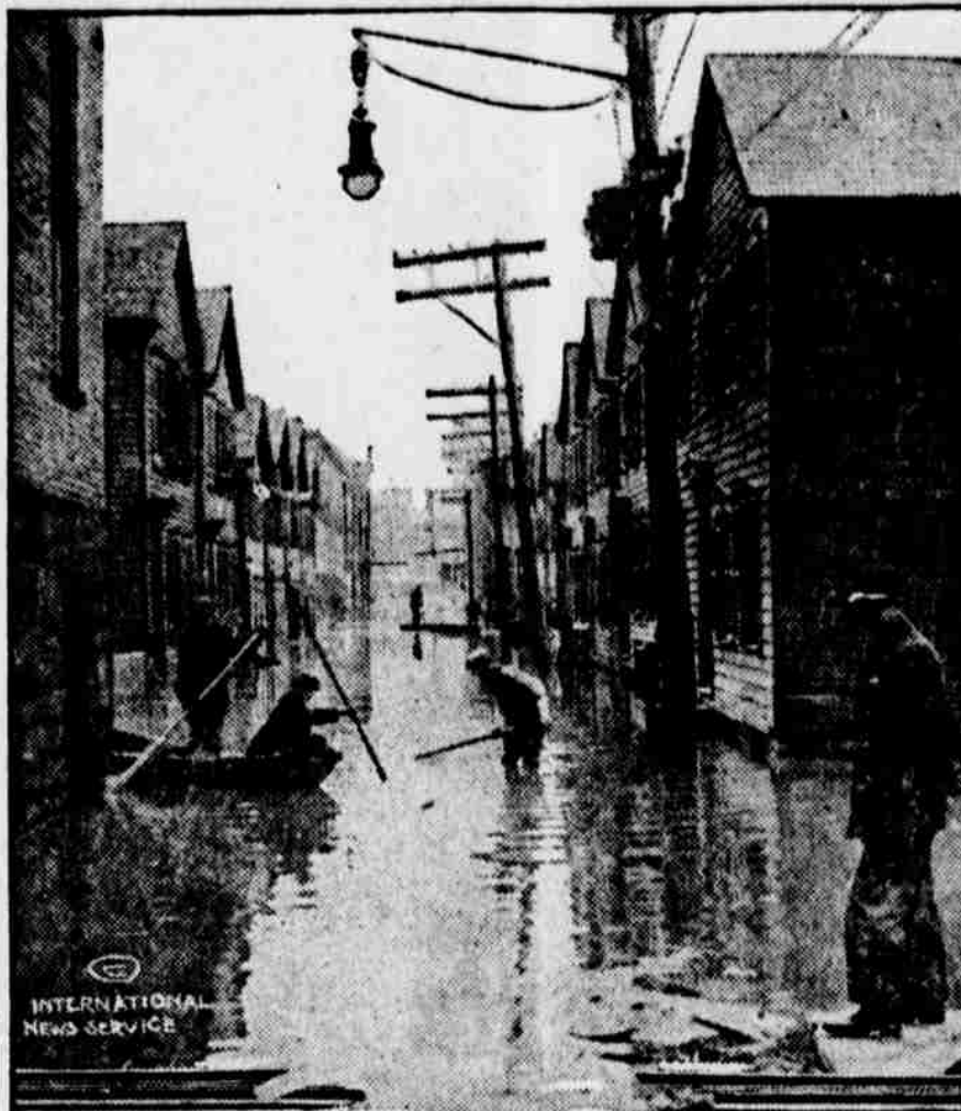
Many cities and towns in the northern part of New York suffered severely during the recent floods. This photograph shows how the people of Schenectady were compelled to make use of boats in the streets.
