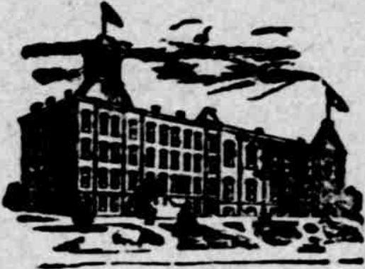
Main Building, 150 Feet Front
