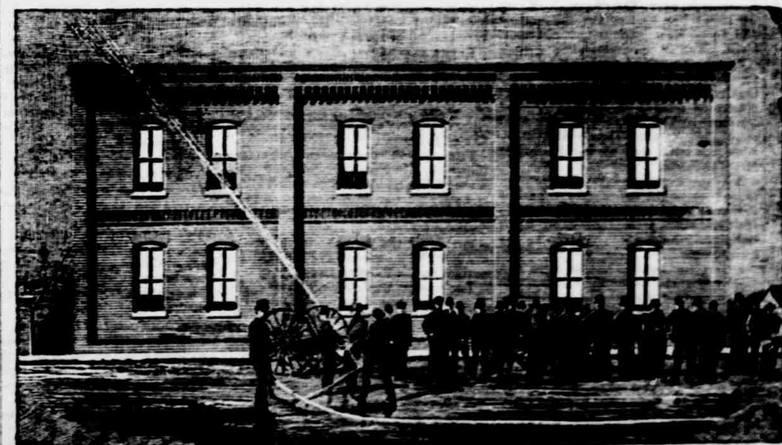
I. O. F. HALL AND FIRE DEPARTMENT HEADQUARTERS.
