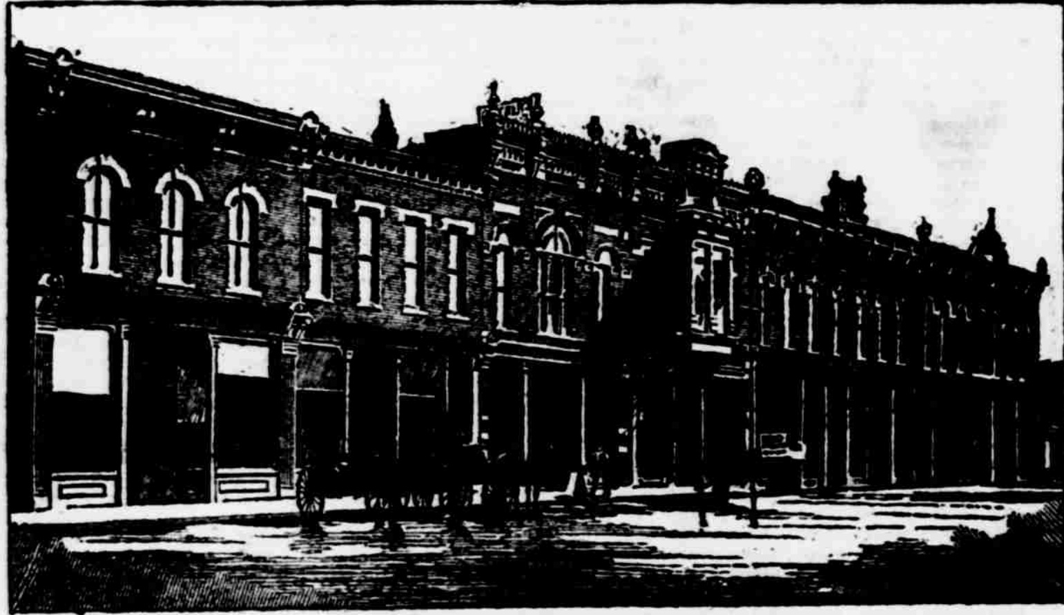
WIENER BLOCK FACING EAST.
