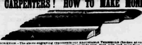
Dascription - The above engraving represents our Adjustable Transmold (broken at one end). It is the only thing in the world that will positively exclude rain, dust, cold and snew from coming under the door. The parts marked A are made of ash, and are united by a strip of heavy, pure rubber marked B, which is adjustable. Its durability has been tested for years. Builders all indorse it.
