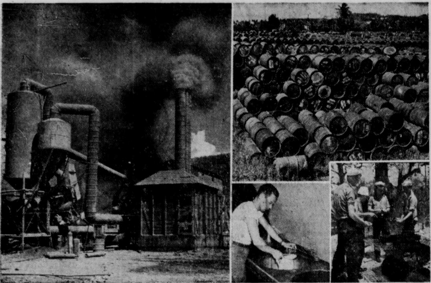
How empty oil drums are being used in the Pacific area is shown by these photos. Left, the drums were used in asphalt plant, as stacks, etc. Center, household use, wash sinks made from drums. Upper right, view of one of the oil drum farms. Lower right, used for barbecue. Other uses include bomb shelters, gateway arches, legs for water tanks, incinerators, sewer pipes and reflectors on light poles.
