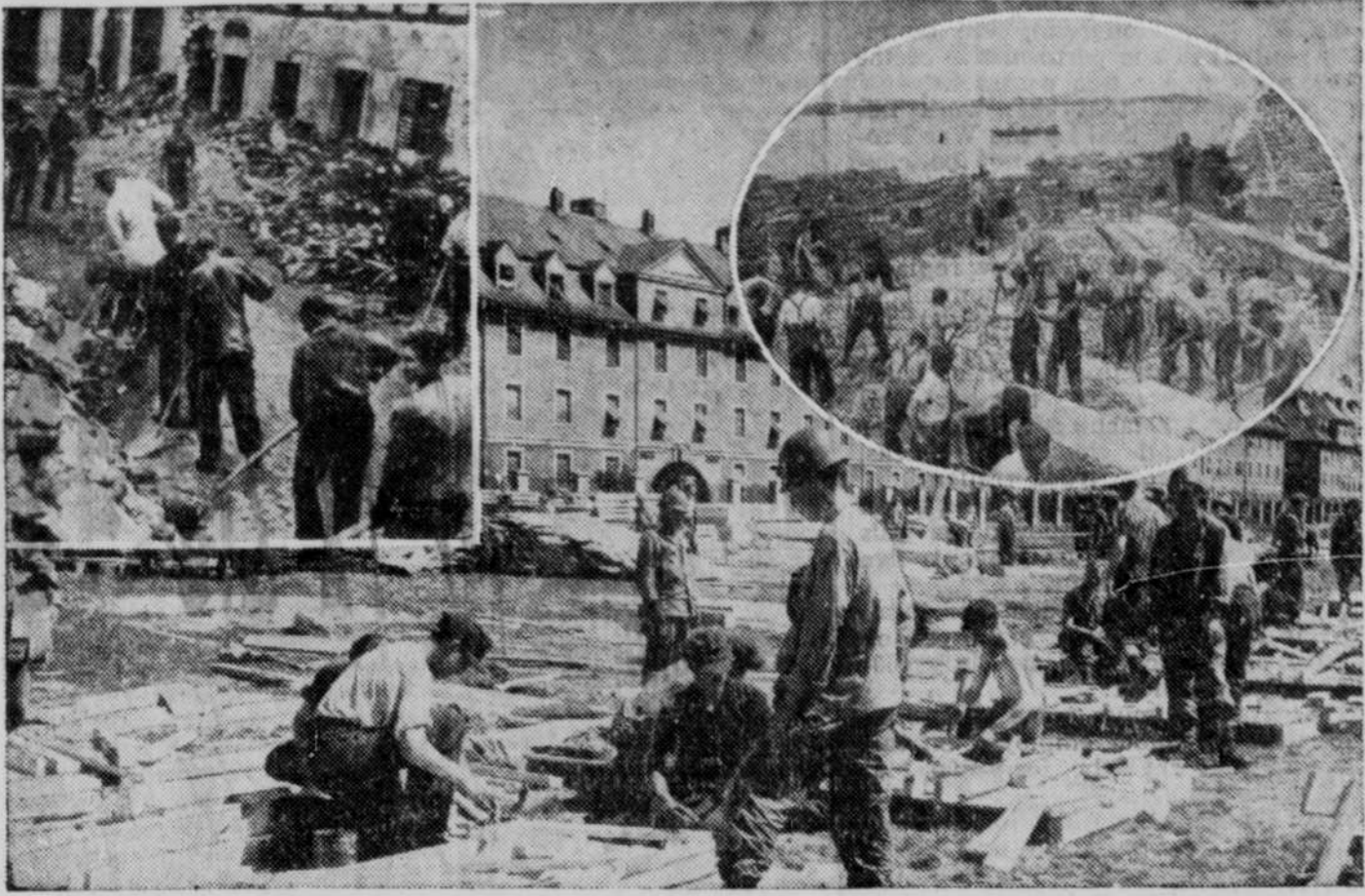
German prisoners, both war and civilian, are put to work as punishment for infraction of Allied military government regulations. They are forced to clean up wrecked buildings and to build beds for returning troops and civilians. At the Citadelle of Port Louis, Lorient, France, they uncovered mass graves of French civilians murdered by Nazis. Picture shows (inset, upper left): German prisoners cleaning up a street in Kitzinger, Germany. Oval: Uncovering a mass grave. Center: An assembly line at Munich making beds.
