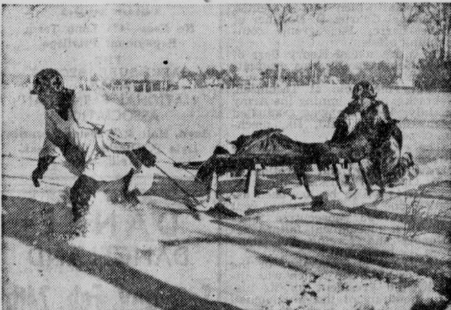
American soldiers fighting on the Western front found that conveying wounded buddies over the snow-capped terrain was a problem until a ski-litter was constructed by Sgt. Waldren Bliss, foreground. Assisting Bliss, in rear, is S/Sgt. George W. Stafford of Petersburg, Va. Many lives were saved by the use of the ski-litter in this section.
