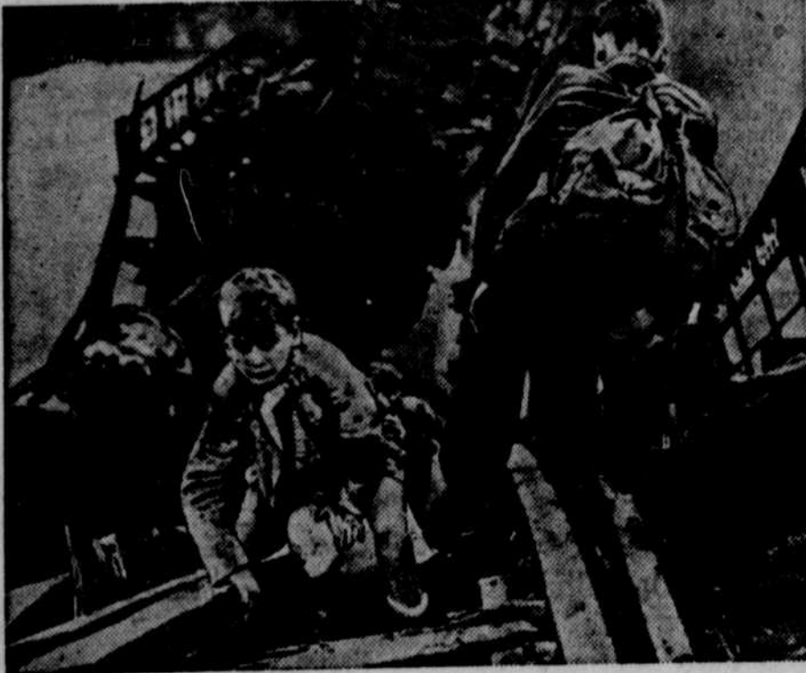
As train lies at bottom of Moselle river after plunging through wrecked bridge, French youth scramble over debris to salvage food from cars.
