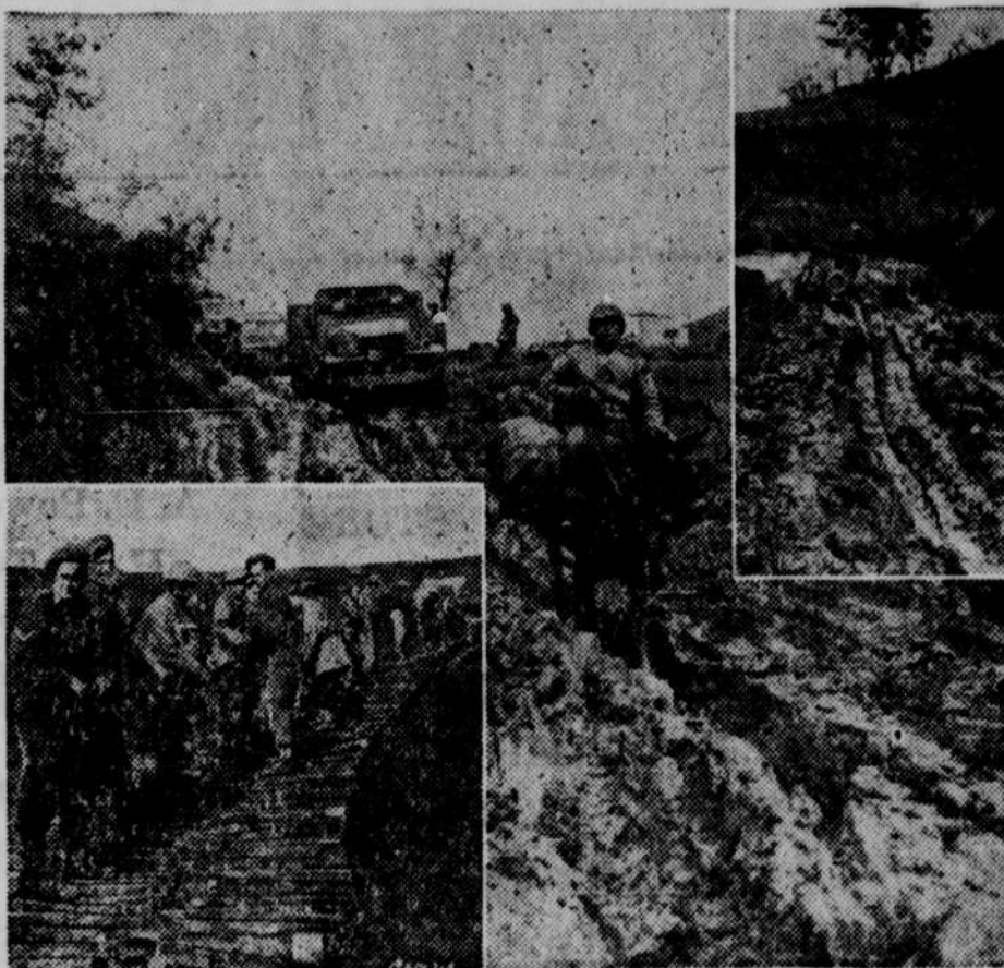
South African troops in Italy have built this road (lower left), out of 105-mm. shell cases, in order to pull their 40-mm. Bofors over it for the Fifth Army. Center—Mules are used to carry supplies south of Bologna when the mud gets knee-deep. Upper right—Hub-deep with mud, the Italian roads have slowed down supplies. In many sections it is necessary to fly in almost all material on account of impassable roads. Thousands of miles of roads are now being constructed by American engineers in France and Italy. While the construction takes time, many of the new roads are in operation.
