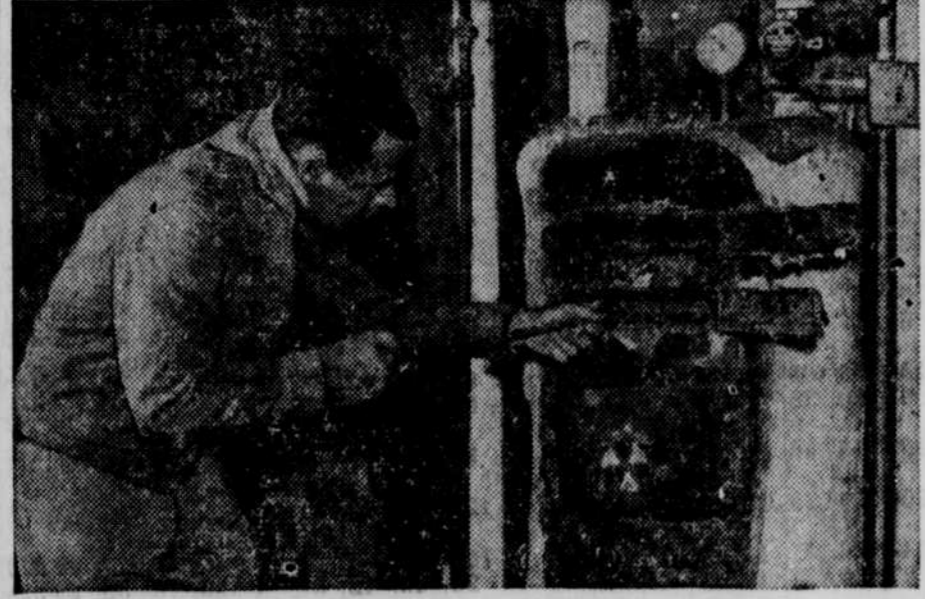
HAVE YOUR FURNACE thoroughly cleaned at the beginning of the cold season. You can do this yourself with a stiff wire brush.
