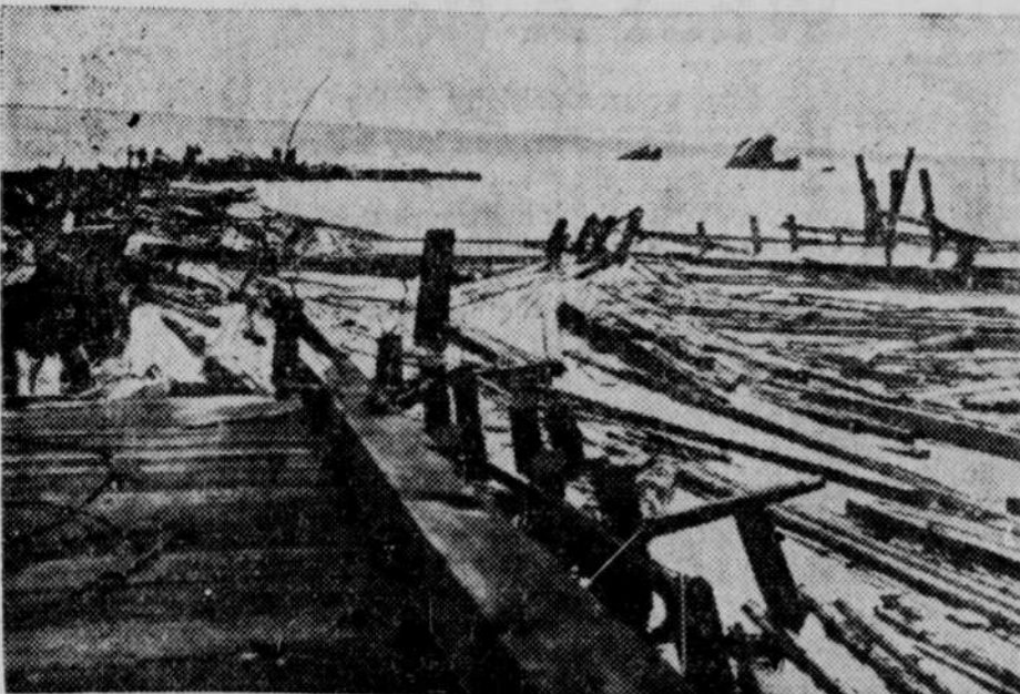
Photo taken at the Port Chicago pier, near Martinez, Calif., where two Liberty ships loaded with ammunition exploded causing loss estimated at 320 lives, only a few bodies of which have been recovered. Wreckage of the pier is shown here, as well as the remains of the vessels, in upper right.
