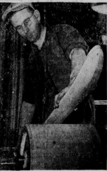
Top: This man, at a Laconia, N. H., ski manufacturing company, is smoothing a ski on a pneumatic drum. Right: With a new ski held in a bracket, this man is sitting on one end to test for flexibility.
