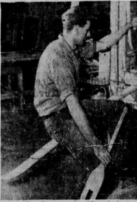
Top: This man, at a Laconia, N. H., ski manufacturing company, is smoothing a ski on a pneumatic drum. Right: With a new ski held in a bracket, this man is sitting on one end to test for flexibility.
