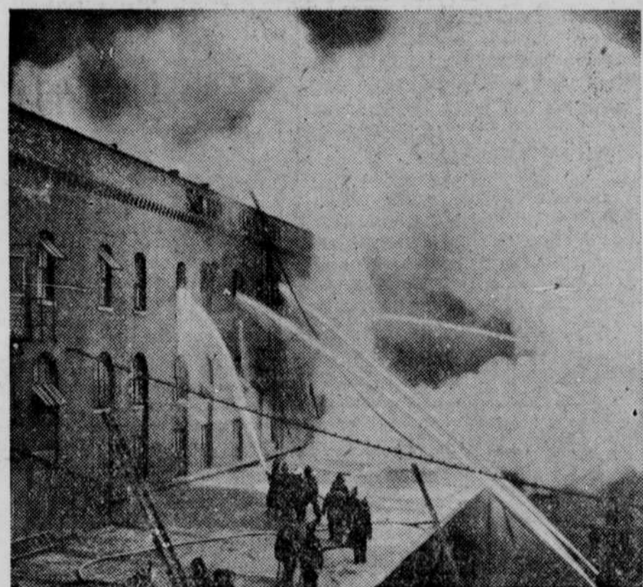
Flames which swept over a block-square building of one of the major meat-packing plants in the Union Stock yards at Chicago caused damage in excess of $200,000. Nearly a third of the fire-fighting apparatus of the city was called to the yards to prevent a spread of the conflagration. Picture shows firemen fighting the blaze.
