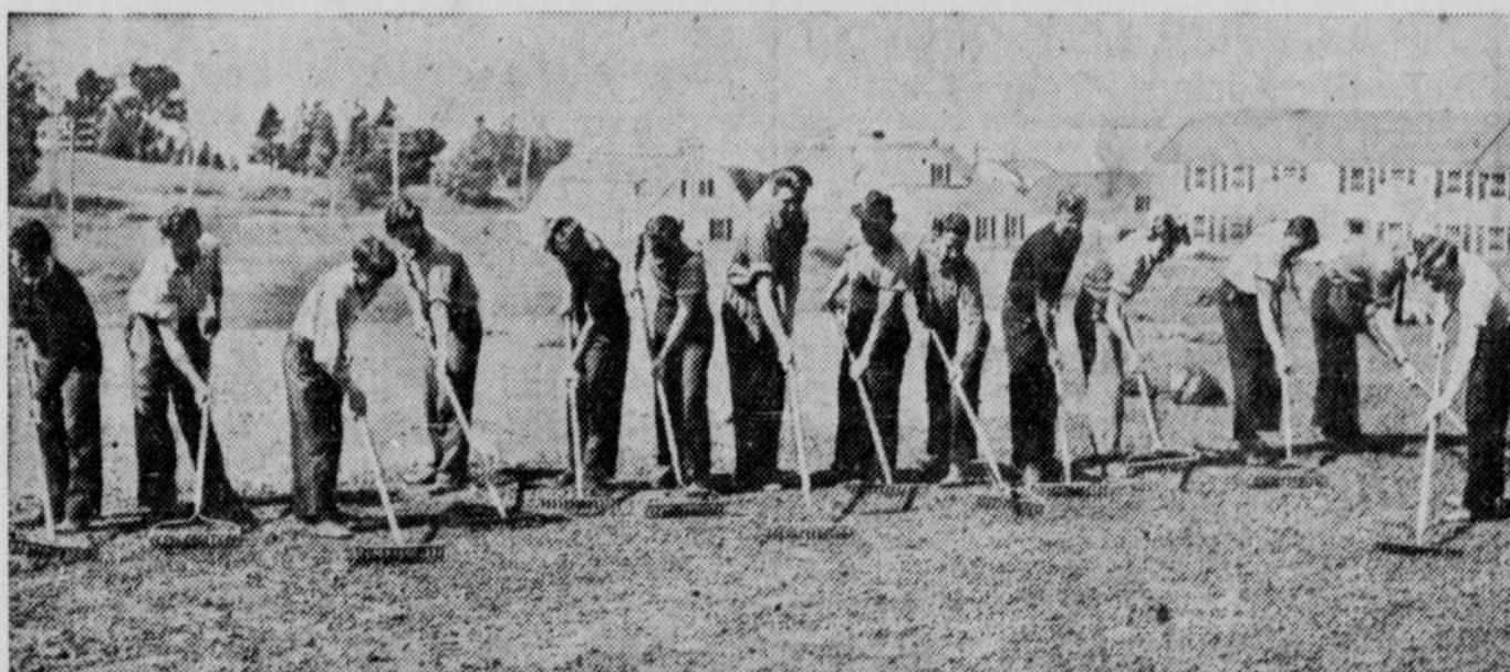
A grading crew of boys, members of the National Youth administration, at work on the new baseball diamond which will be used this summer for camp games at Quoddy Village, Eastport, Maine, the model community of the suspended $36,000,000 federal Passamaquoddy bay tide-harnessing power project, which has been taken over by the N. Y. A. for the purpose of vocational training.
