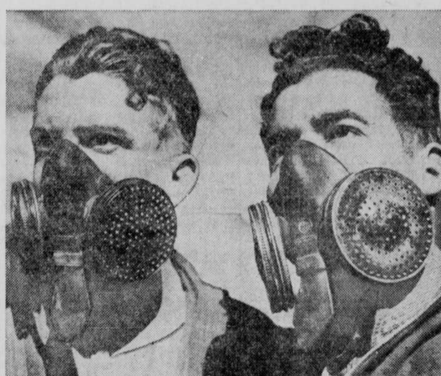
Not for deep-sea diving and not for service in the Spanish war, are these odd appliances that these men wear. They are to be used for construction work on a new road to the national park at Yosemite, Calif., and are dust masks which will prevent inhaling rock particles.
