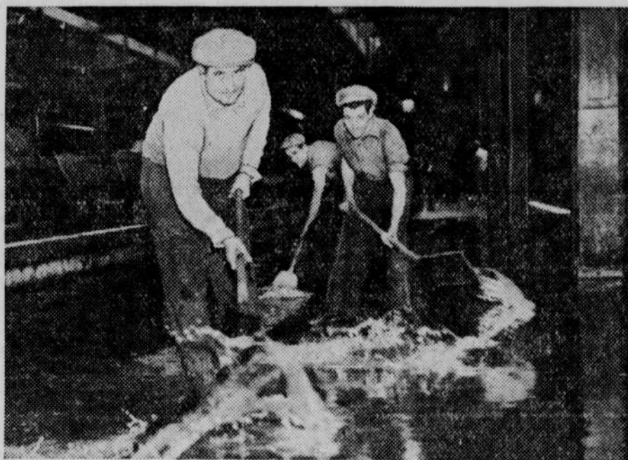
Photo shows workmen trying to clear tracks at the Union station in Chicago of a flood estimated at three to ten feet deep. A 36-inch water main burst putting 14 railroad tracks out of commission. The water also flooded portions of the new post office. Passengers from suburban trains were forced to alight from inbound trains about five blocks from the station. Damage was estimated at $200,000.
