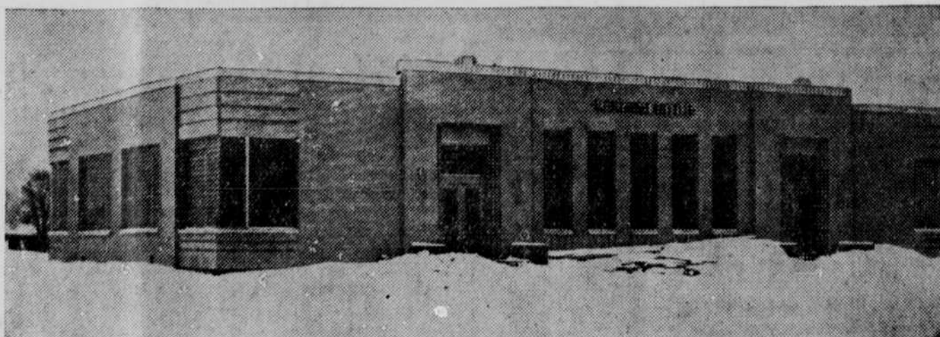
Exterior view of the new Park school in Hibbing, Minn., showing areas of vacuum glass brick replacing the usual windows. This new kind of construction has earned for this novel structure the title of the "Glass" schoolhouse.
