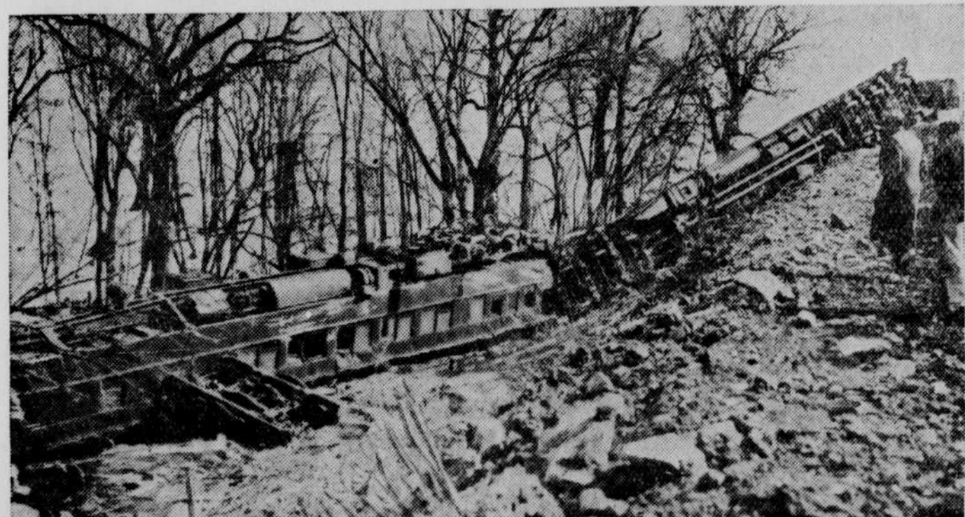
When this Rock Island passenger train, bound from Chicago to Kansas City, left the rails near Excelsior Springs, Mo., and rolled down a 30-foot embankment, fortunately not a single passenger was injured. Three Pullman cars and one diner went into the ditch, and the only person hurt was a brakeman
