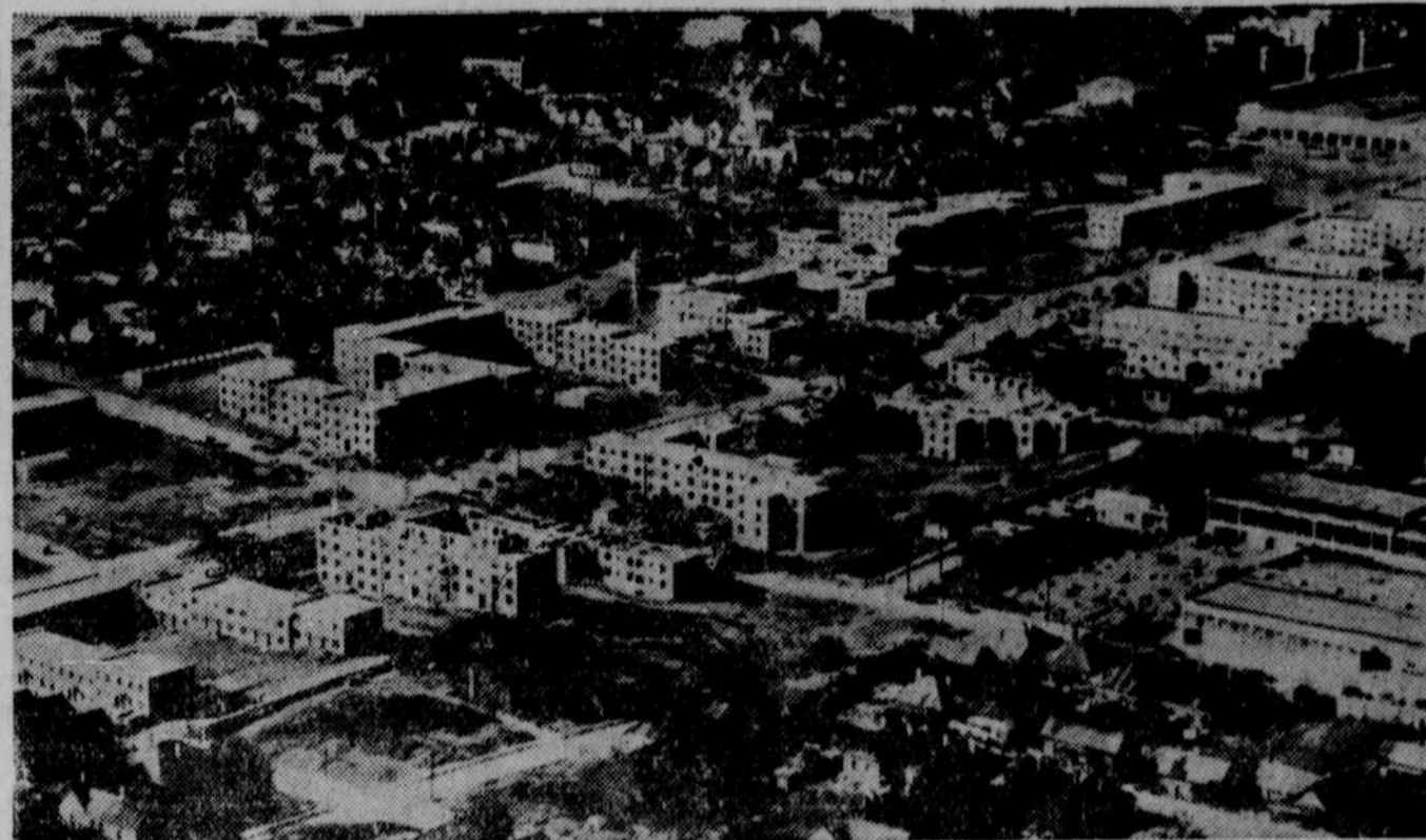
Aerial view of the PWA's $2,875,000 Techwood housing project in Atlanta which President Roosevelt helped to dedicate by the unveiling of a commemorative plaque. The project will house 600 families.
