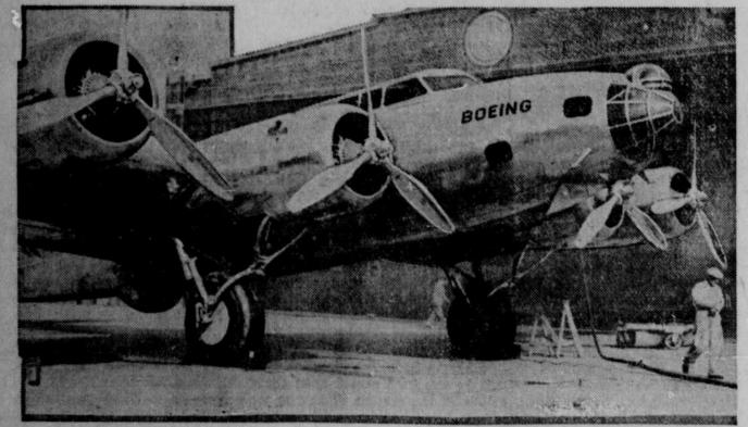
After a year of secret operating this greatest bombing plane in the world, the Boeing 230, was completed for the army air corps at Seattle and appeared for test flights. It has four 700-horsepower motors, a wing spread of more than 100 feet and is 70 feet long. Its weight is about 15 tons and its expected speed 250 miles an hour.
