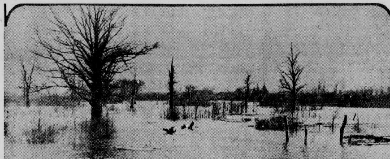
Paul road, usually a well-traveled thoroughfare, takes on a desolate appearance after the overflow of Black creek inundated a large area at Chill.
