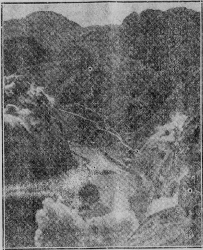
If this picture were wired for sound, you'd hear a pandemonium of noise as if the sky were falling on you. The photo was made at the exact instant that several charges of explosive were touched off in the Black Canyon, Boulder City, Nev., blowing thousands of tons of rock into the Colorado River, thereby diverting the course of the stream into a tunnel prepared for it through a mile of mountain. This was the first important engineering step in the construction of Hoover Dam, the largest project of its kind ever attempted.
