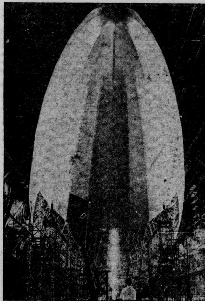
Work is progressing rapidly on the new Navy dirigible, U. S. S. Macon at Akron, Ohio. This photo, made in the giant hangar where the big craft is nearing completion, shows the nose of the Macon after it had been covered with fabric. Although she will be a sister ship to the Akron, the Macon is much larger than the former.
