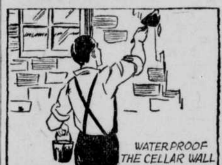
WATERPROOF THE CELLAR WALL
