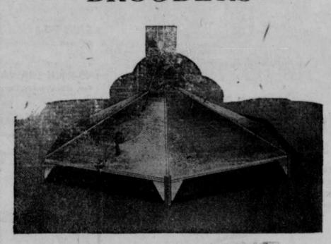
As in all Jamesway Brooders, much practical research and testing have gone into this gas-burning unit. Extremely simplified in design and equipped with controls that give it a high degree of economy and dependability. Operates on manufactured, natural or bottled gas. Complete with 72-inch hover for 500-550 chicks. Weighs 85 pounds.
