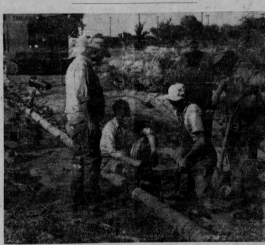
Crossing river with pipeline is not an easy task. Dewatering is done through a surface pipe with suction through vertical pipes. William Barnett, Omaha Negro (extreme right), is a novelty to O'Neill youngsters. . . the only colored man in town.
