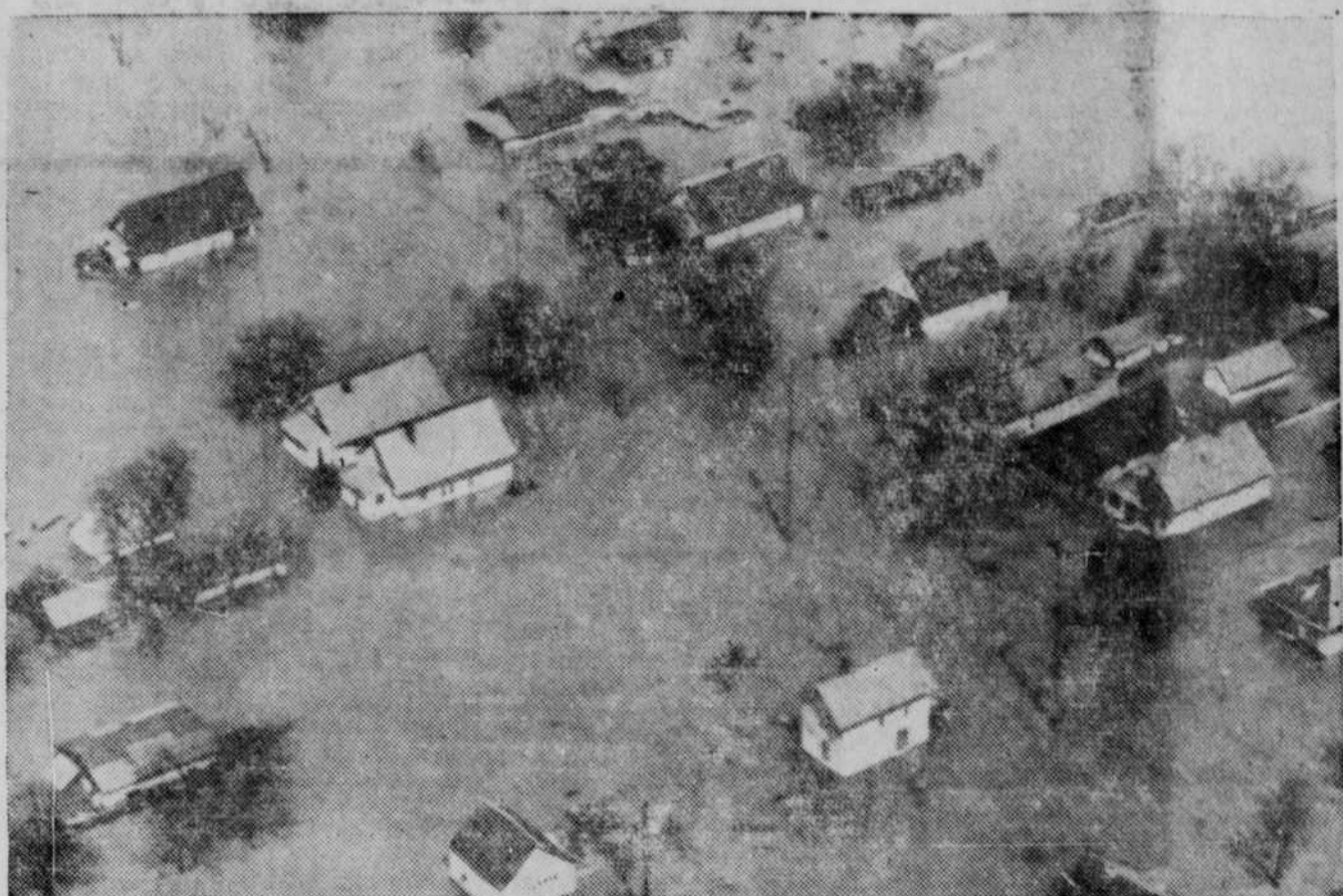
FLOOD SWEEPS LANSING
