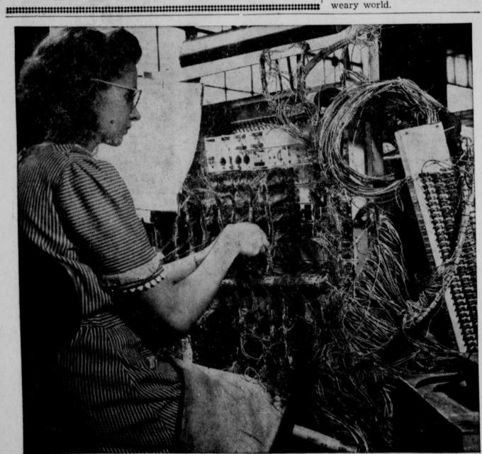
"ONE AT A TIME" IS THE RULE when connecting by hand the thousands of wires on new tele-phone equipment. Since the load on present equipment has reached the absolute limit and more switching equipment is needed to provide normal service, work is being rushed on all kinds of costly telephone facilities. Soon this switchboard can share the service burden and help reduce delays that may arise from present overloads
