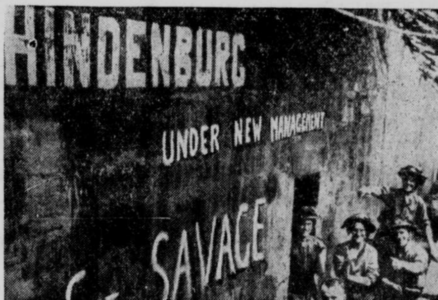
"Hindenburg Bastion," as this captured German "West Wall" concrete emplacement was known, is the present abode of Sergeant Savage and his Chindits. The new occupants, shown pointing to a comment on the wall, are members of a Bofors gun crew.
