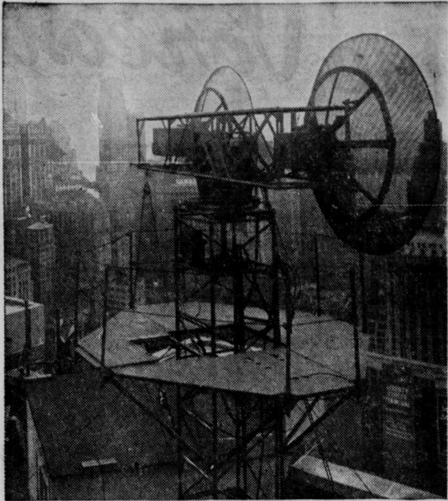
Shown atop the New York telephone building are the antennas used during demonstration of a secret army radar microwave relay system. The demonstration, conducted by Bell telephone laboratories, included a two-way voice transmission carried out successfully over links totalling 1,400 miles. It was announced as entirely practical and successful.
