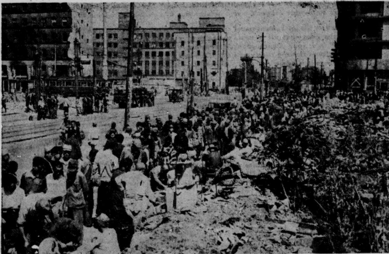
Customers crowd around the sidewalk stands in the Ginza District in Tokyo, which is similar to New York's Fifth Avenue. Shopkeepers, their stores destroyed by bombs, set up their wares in the street, and carry on their business outside the wrecked buildings. In the background is the famous Jap Department Store, Takashimaya, where only two floors are now in use.
