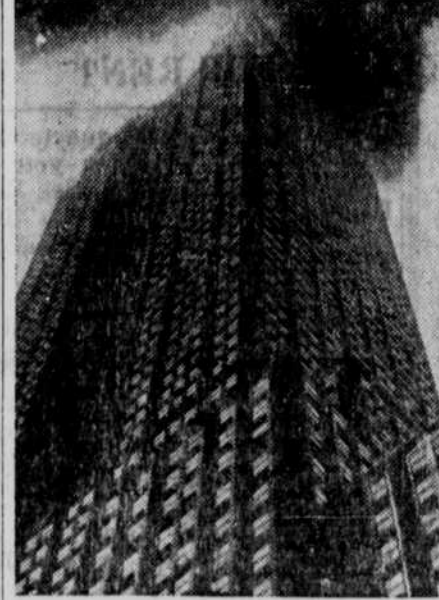
The tower of the Empire State building, world's tallest, is shown enveloped in fog, smoke and flame after a U. S. army B-25 bombing plane crashed into the building recently.
