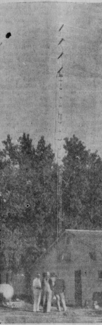
Jacobson-Beha tower . . . overall height 62 feet.
