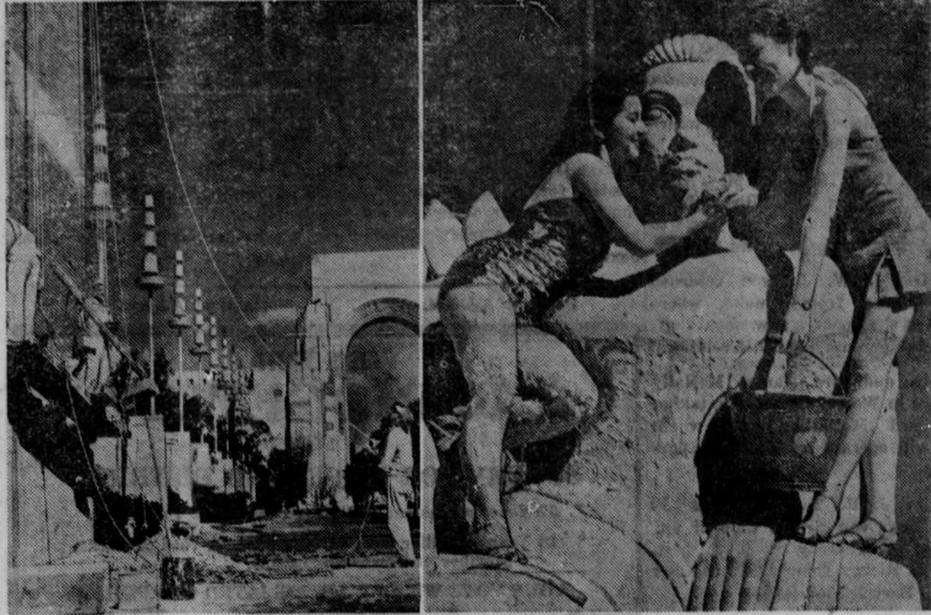
Face-lifting operations for the 1940 Golden Gate International exposition are well under way in preparation for the opening day, May 25. Left: Workmen are pictured plastering and painting in Treasure Island's court of reflections, where an entirely new color scheme will greet first-day visitors. Right: Statuary gets a bath on the exposition grounds. Jeanette Adams and Fay Lacey do their share with this sculptured figure.
