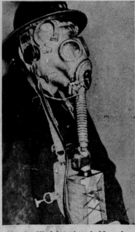
Smoke-filled interiors hold no fear for fire laddies equipped with this combination gas mask and telephone. The mask protects the fireman as he 'phones directions for fighting a stubborn blaze.
