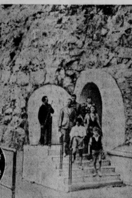
FOR HOSPITALS —Here is harbor entrance to Ramsgate, England's new subterranean hospital.
