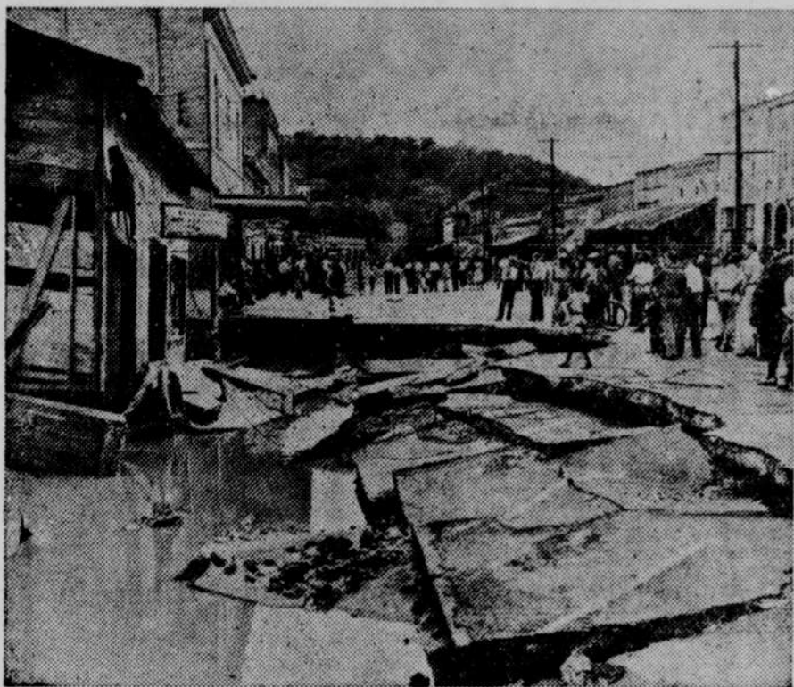
Undermined by flood waters from a swollen tributary of the Alabama river, this section of the Prattville, Ala., main street collapsed, halting traffic through the business district. Floods were caused by heavy rains, and though there was no loss of life, more than 3,000 persons in the southern part of the state were forced to flee their homes.
