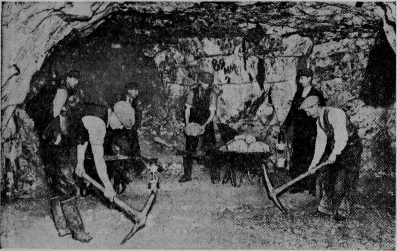
Under the town of Chiselhurst, Kent, England, stretch 22 miles of caves hewn out of chalk by the early Britons when they sought protection from the Roman invaders. The caves are now being converted into air-raid precaution shelters, fitted with all modern devices for protection. Four to five thousand people can be accommodated in the 2,000-year-old caves.
