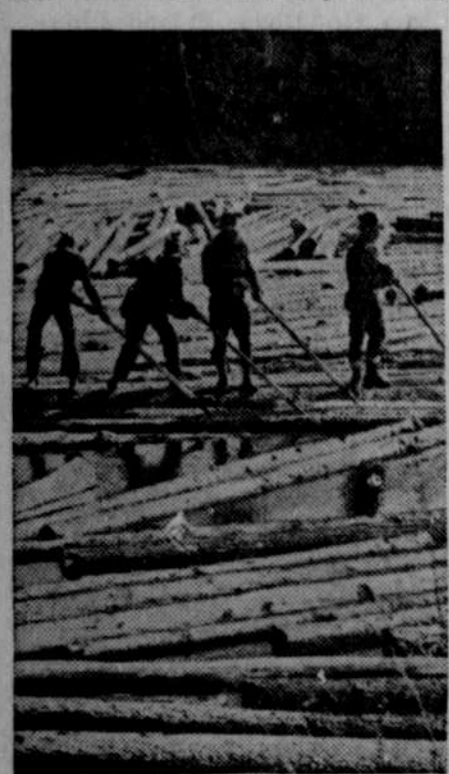
After the spring breakup in Maine, logs are drifted down rivers to the saw mills. It's the job of these log rollers, with caulked shoes, to keep the lumber moving.
