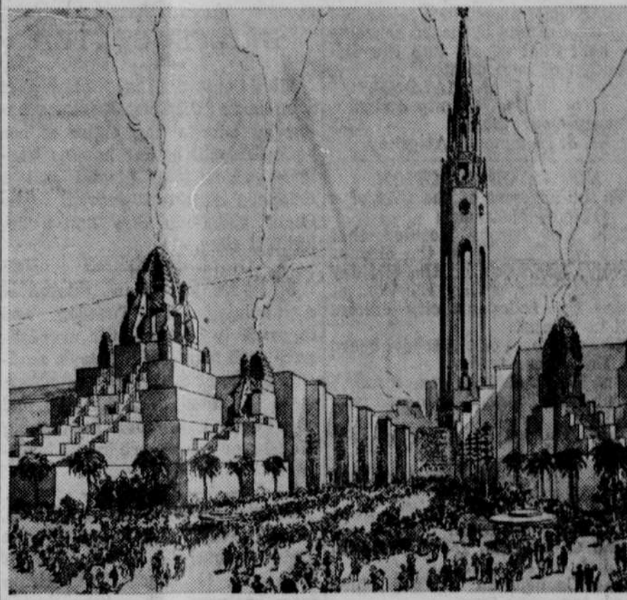
Main entrance gates of the 1939 Golden Gate International exposition on Treasure island in San Francisco bay where millions are expected to enter next year are shown in this sketch by Artist Louis Rothe. Towering above the exposition is the 400-foot Tower of the Sun.
