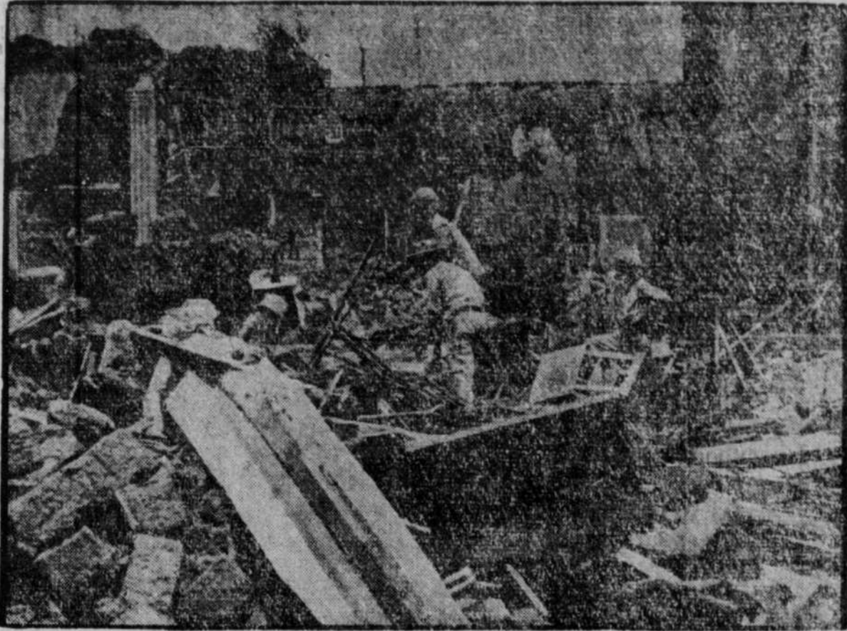
This picture graphically tells the story of the earthquake and resultant fire that took a toll of more than 2,000 lives and untold property loss in Nicaragua. Above is a typical scene in the once fair city of Managua, where natives search for remnants of their belongings in the ruins of their homes. United States Marines are aiding gallantly to alleviate the sufferings of the people.
