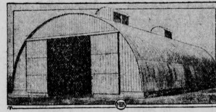
This building isn't a hangar for a baby plimp. It's a new type farm ouilding appearing in the Middle West for storing grain and large farm machinery. It is supported by fabricated steel trusses 15 feet apart. It is 40x90 feet, and is said to provide the largest storage space with the least expense and with the greatest strength against wind stresses.
