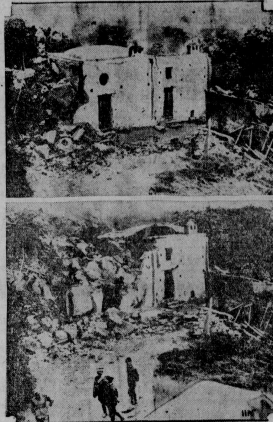
Above is a typical home in the peaceful little town of Terzigno, Italy, with the ever-threatening Mount Vesuvius in the background, while below is the same house in a mass of ruins after being engulfed by the swiftly moving red-hot lava during the recent violent eruption of the volcano. Considerable damage was done in the surrounding country and the loss of life was tremendous. (International Newsreel)
