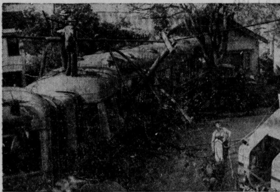
After hitting a piece of concrete on the rails, this train jumped its tracks, crashed into a steel trolley pole and careened 30 feet across a street, stopping only two feet from the home of Oscar Houman. He later said he thought the noise was an earthquake. The accident occurred in Berkeley, Calif. Seven passengers received minor injuries.
