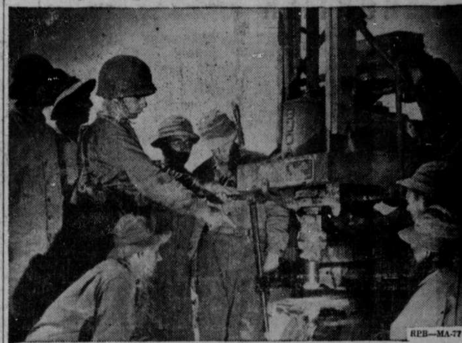
The best engineering equipment in the world is at the disposal of the U. S. Army Corps of Engineers, including lots of special-purpose machinery that's going to help in building the postwar world. The earth auger shown in the picture above is one of the machines the Engineers use to build and fight.
