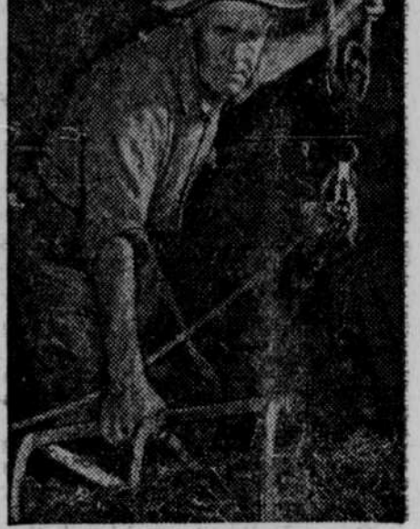
Ropes running through pulleys should be reversed end for end to equalize wear. (Picture from U. S. Soil Conservation Service.)
