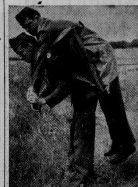
One man can carry a casualty with this new type litter invented by Lt. Col. S. H. Bingham. It can also be adapted for a two-man carry by changing the trap arrangement.
