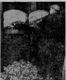
Following sorting and testing, tubes are fed to the furnace. The
