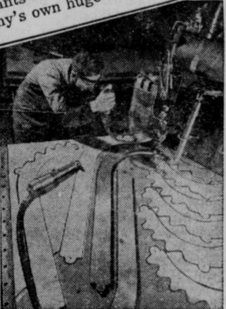
Routing machine (above) uses metal template as guide to make wood patterns. Left: Dorsal fin gives name "Dragon's Teeth" to row of rear sections.
